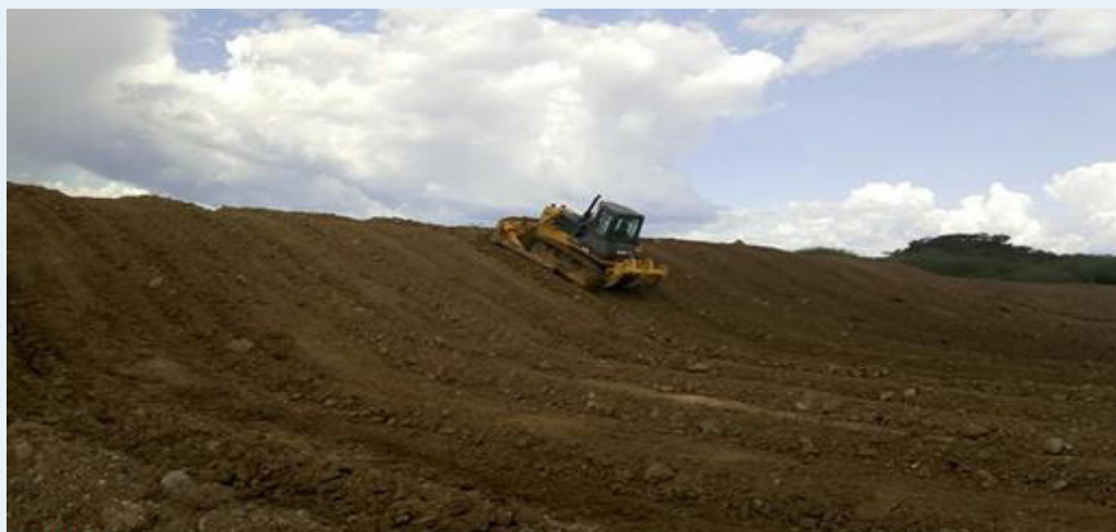
Figure 3.5 Mechanized excavation of water pan
