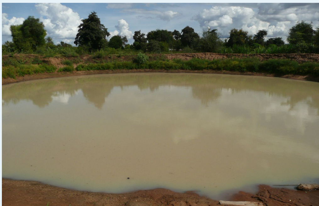
Figure 3.1 A water pan in a protected catchment collects clean water
