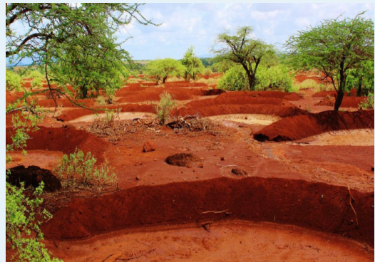
(b) Demi-Lune (Half-moon) design are large semi-circular bunds with a basin utilizing an external catchment or point sources runoff, such as from road drains, foot paths, steep hillsides and extensive open areas.
