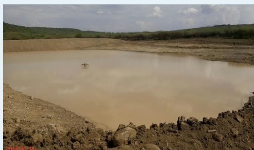
(Photo credit: Baringo WFP-AC project) (a) A newly excavated water pan
