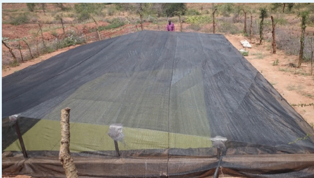
Figure 2.12 Covering the farm pond with shade net
