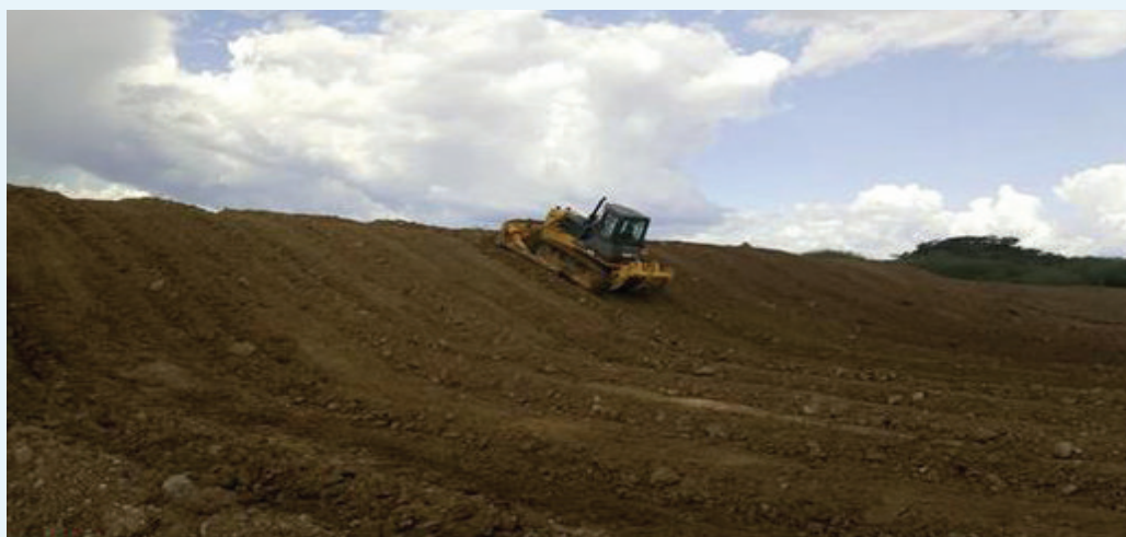
Figure 3.5 Mechanized excavation of water pan
