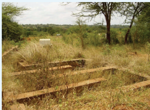
(b) Concrete zig-zag inlet channel
