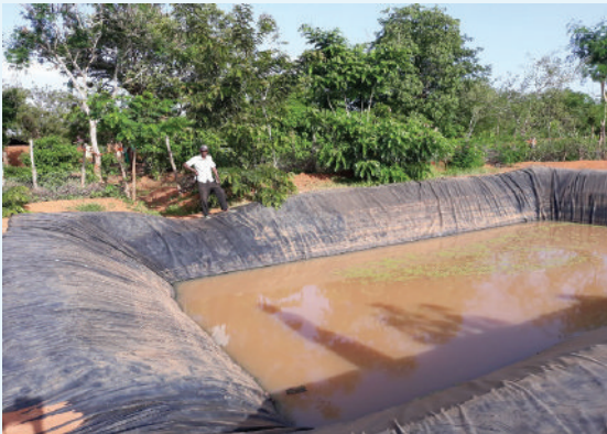
(a) Farm pond lined with dam-plastic material
