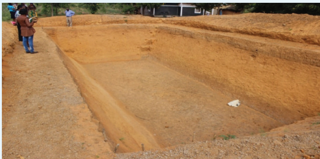
Figure 2.8 Farm pond with smooth side slopes
