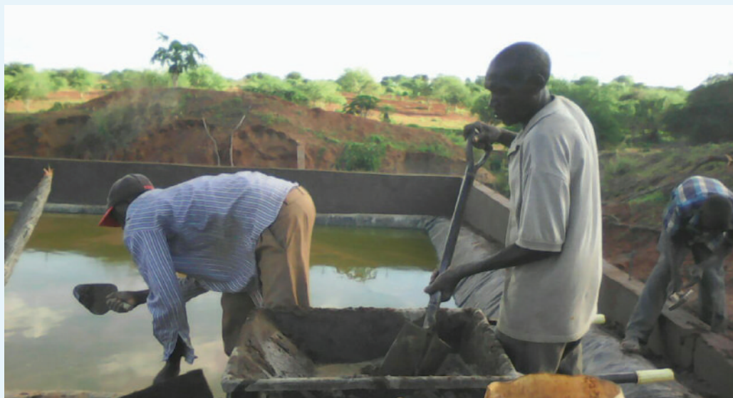
Figure 2.10 Construction of perimeter wall
