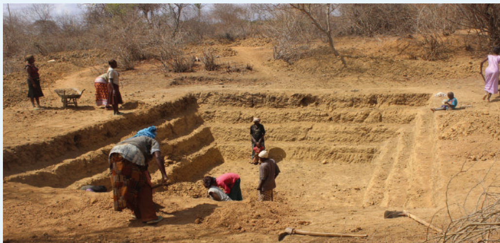
Figure 2.6 Excavating the Farm pond
