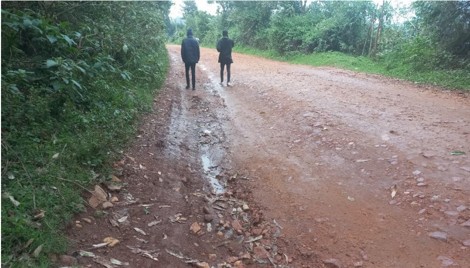
Photo #3: Road Sections Requiring murrum and compaction
